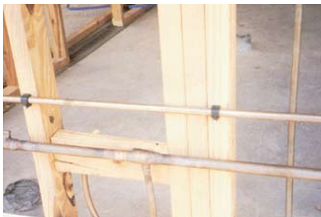
Fig. 14.2 Installed Piping Services Prior to the Installation of Hebel™ PowerPanel™
