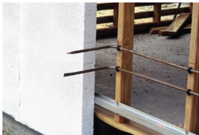
Fig. 14.2 Installed Piping Services Prior to the Installation of Hebel™ PowerPanel™
